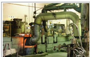
1 Melting 熔化 High-frequency electric furnace 高頻電爐
