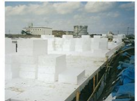
EPS除去作業 Removal of EPS
