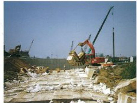
EPS除去作業 Removal of EPS
